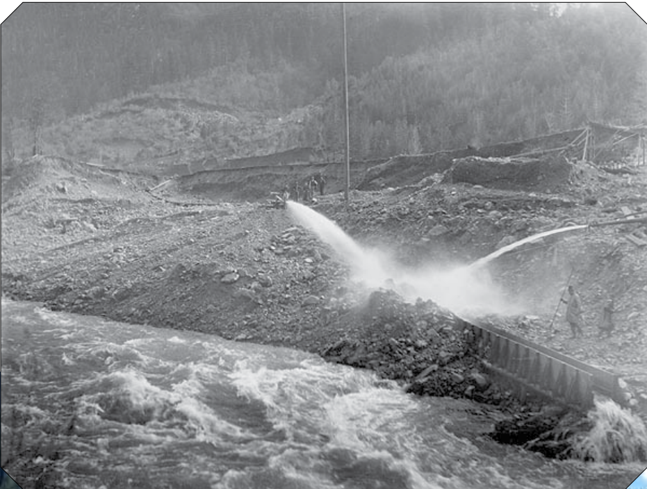
Historic hydraulic mining on the Salmon River -- photo from the Chico State University collection
